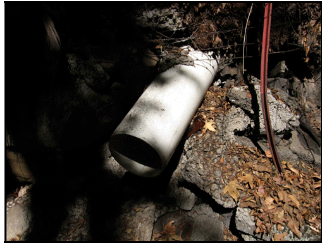
Photo 7 - Worksite 5, view upstream of eroded riprap. Photo 8 - Worksite 6, 12" drainpipe and eroded grout.
