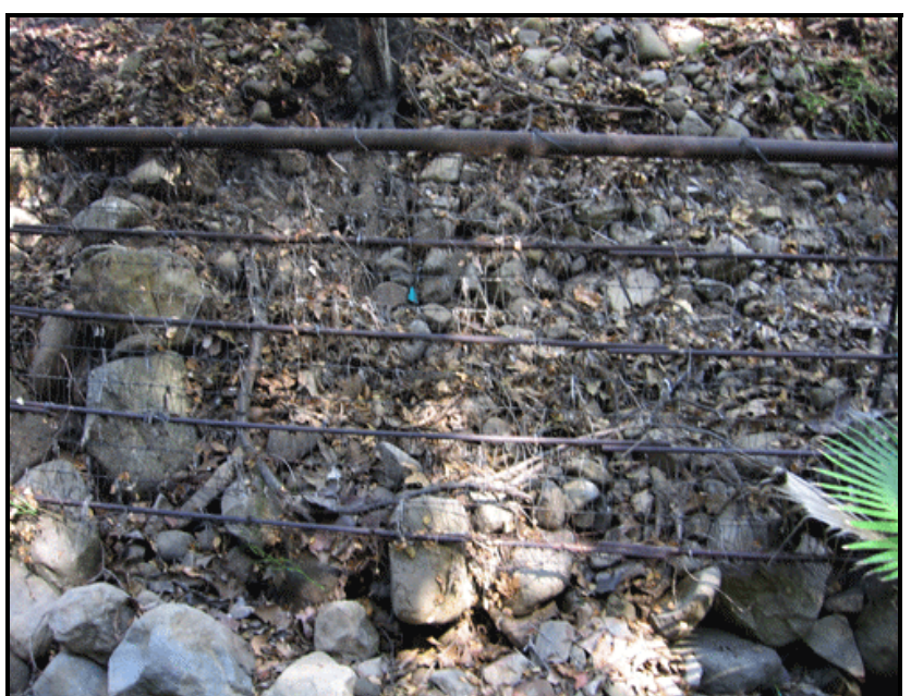
Photo 5 - Worksite 3, view upstream of bedrock. Photo 6 - Worksite 4, pipe and wire revetment.
